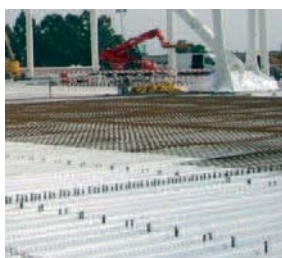
Through deck welding technology in composite construction
